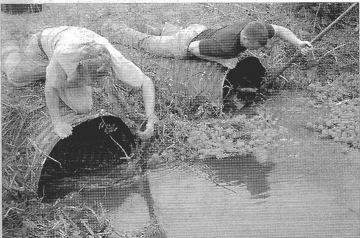
While taking a "break" from work along Woodlands Trail, University of Louisiana Lafayette students decide to restore the flow of water from a drainage ditch near the Woodlands Trail entrance. After removing massive storm debris which restored drainage into Planter's Canal, the water line on nearby trees dropped 15 inches.
